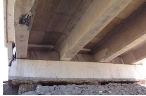
(b) Chada bridge with no diaphragms, Chile
